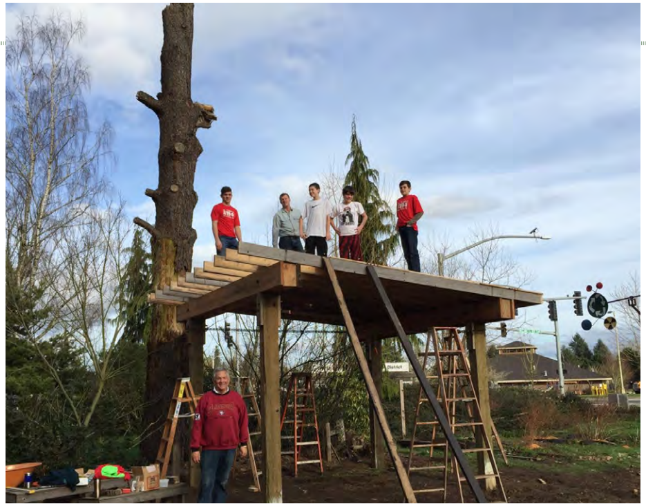
Green roof structure under construction
